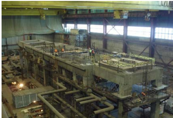
Turbo-unit foundation underpinning
