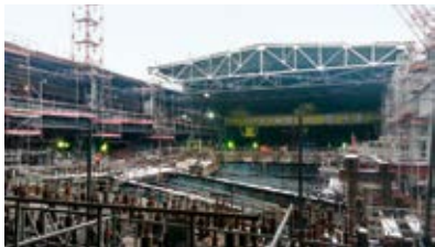
Dismantling of inter-centre sills
