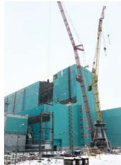
Lifting of an enlarged block of E/17–18 columns
