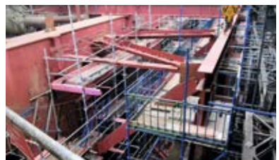
Installation of the retaining under-ridge girder
