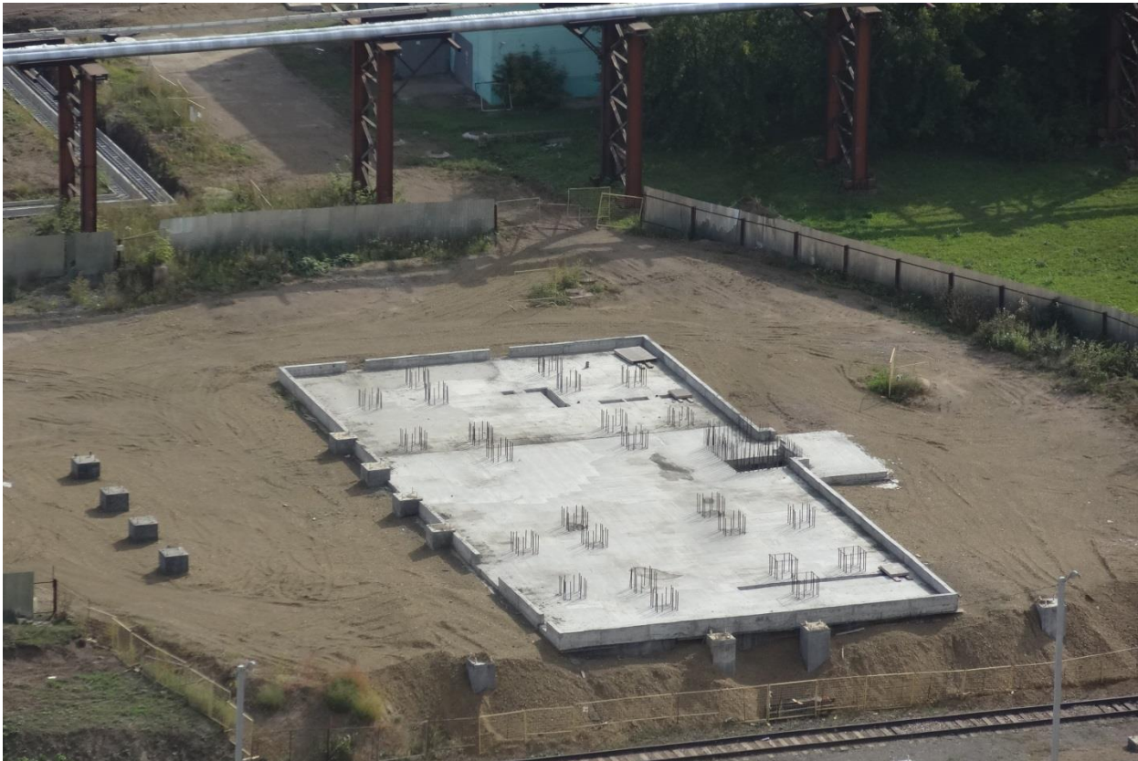
DARS. Foundations for the silo warehouse
