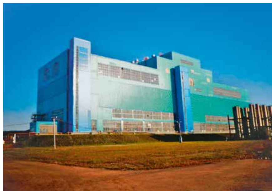
Fuel Receiving Station
